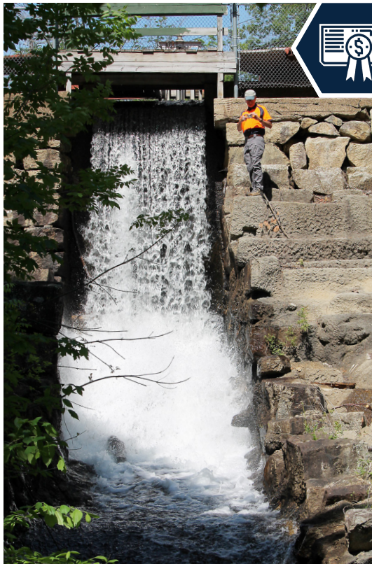
Dan Hole River Dam inspection.
