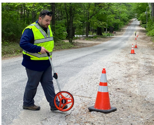
Mitigation and Recovery Chief Austin Brown takes measurements during a PDA in Alton.
